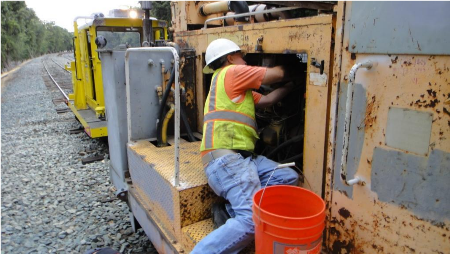
Mike H. modifies the compressed air system on the old-old tamper to accommodate an umbilical hook-up from the Kalamazoo tug
