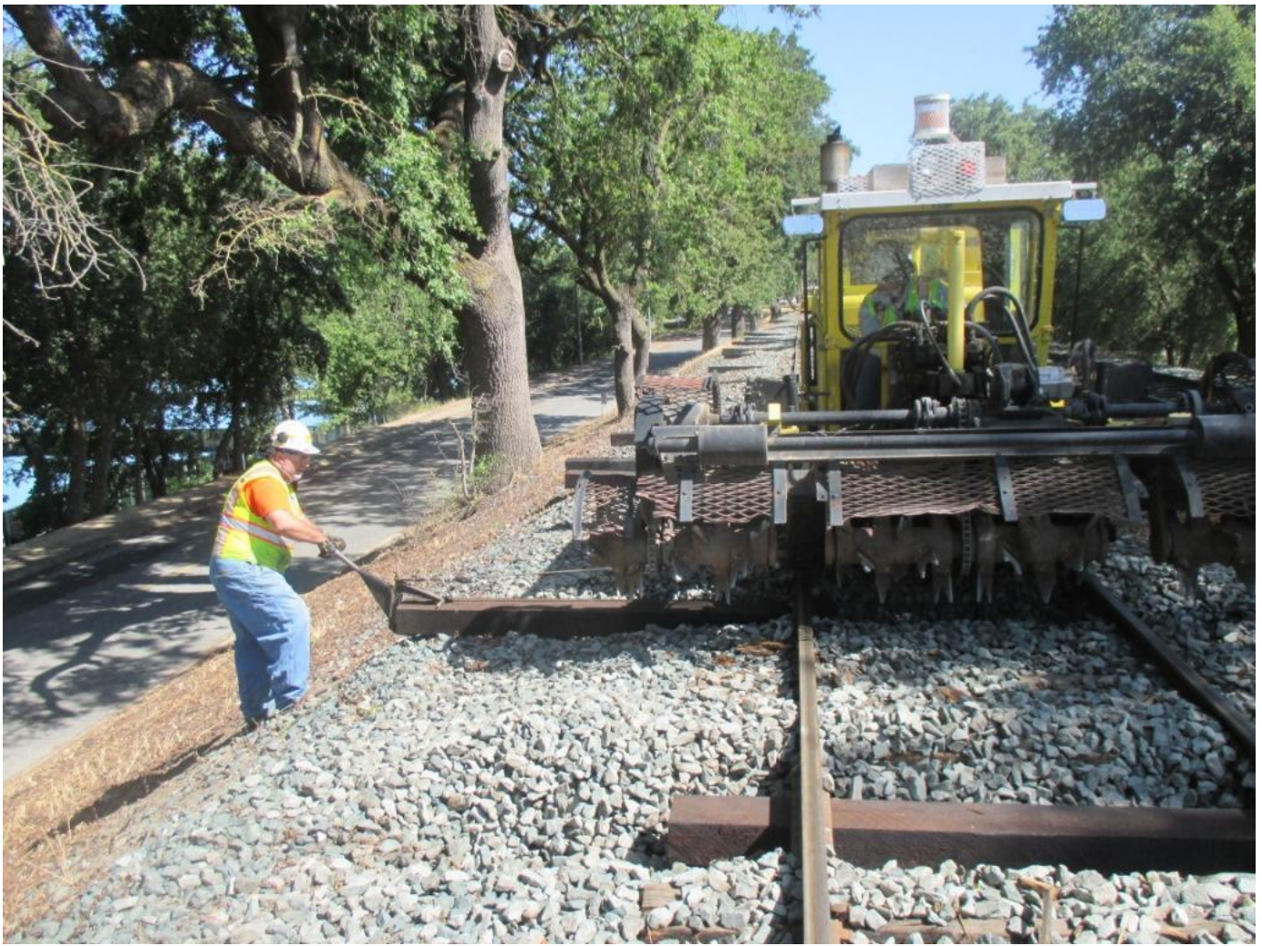
Heather operating the scarifier and Mike F. on the ground pull new ties into place
