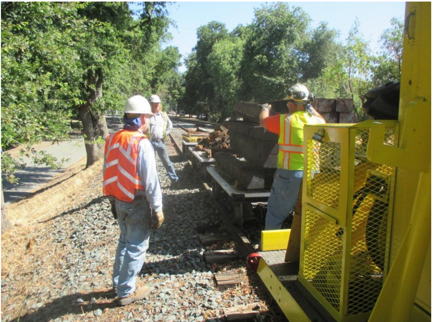
Mike M., Mike F., and Steve roll ties off the flatcar for placement and installation
