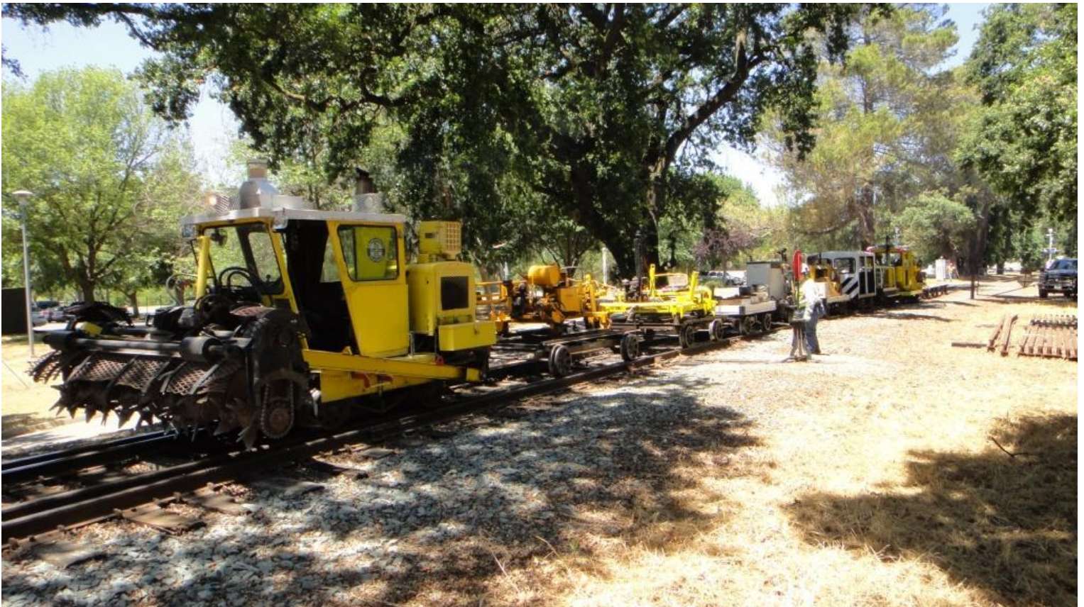
Now, that's an impressive line-up of track machines
