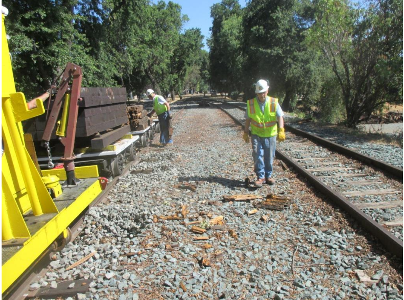
Clem and Mike W. clear out tie debris strewn about the line
