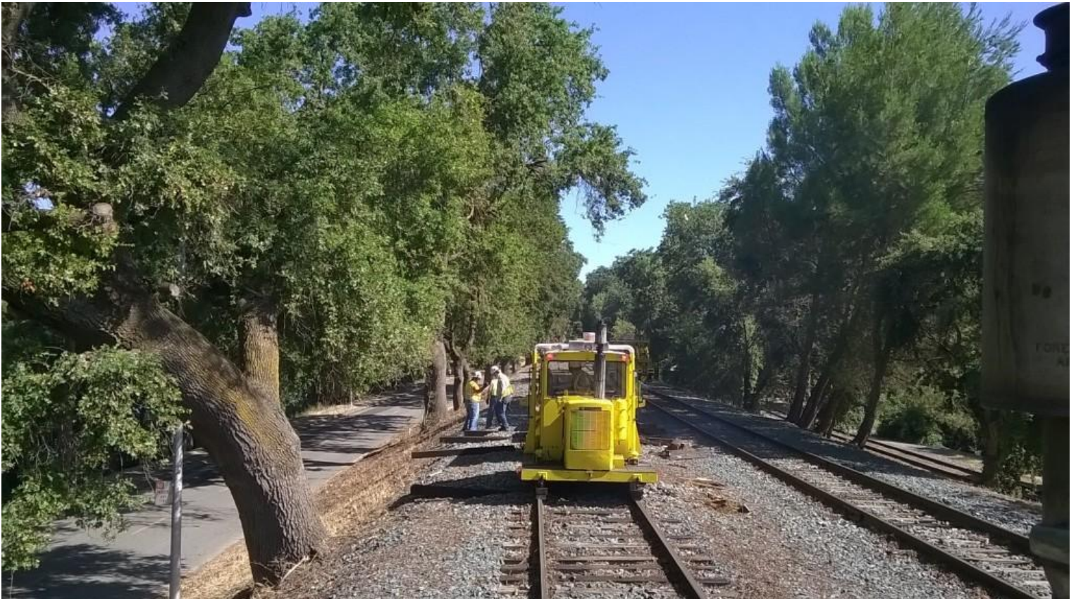
The tie replacement operation is like a production line
