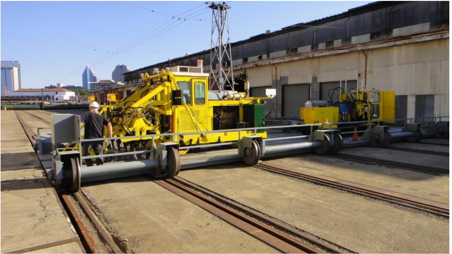
Making room in the Erecting Shop: the new-old tamper and tie-shear on the transfer table
