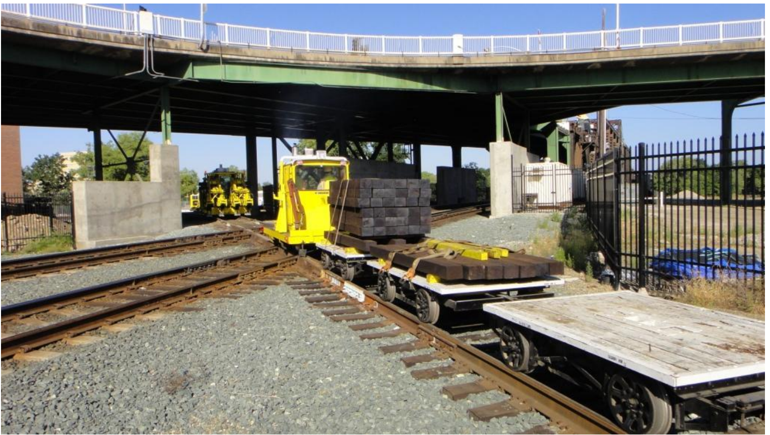
The new-old tamper and Kalamazoo tug pulling tie-laden flatcars crosses the UP Main at RV 988
